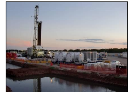
Natural Gas Drilling Rig
