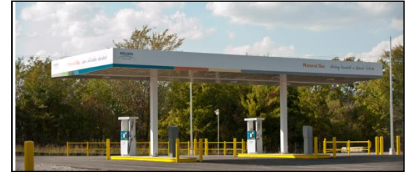
Louisiana CNG Station
