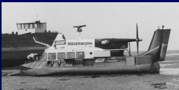
SRN 5 1964 Length 12.7m Width 7m All up Weight 6.6t Payload 2.6t
