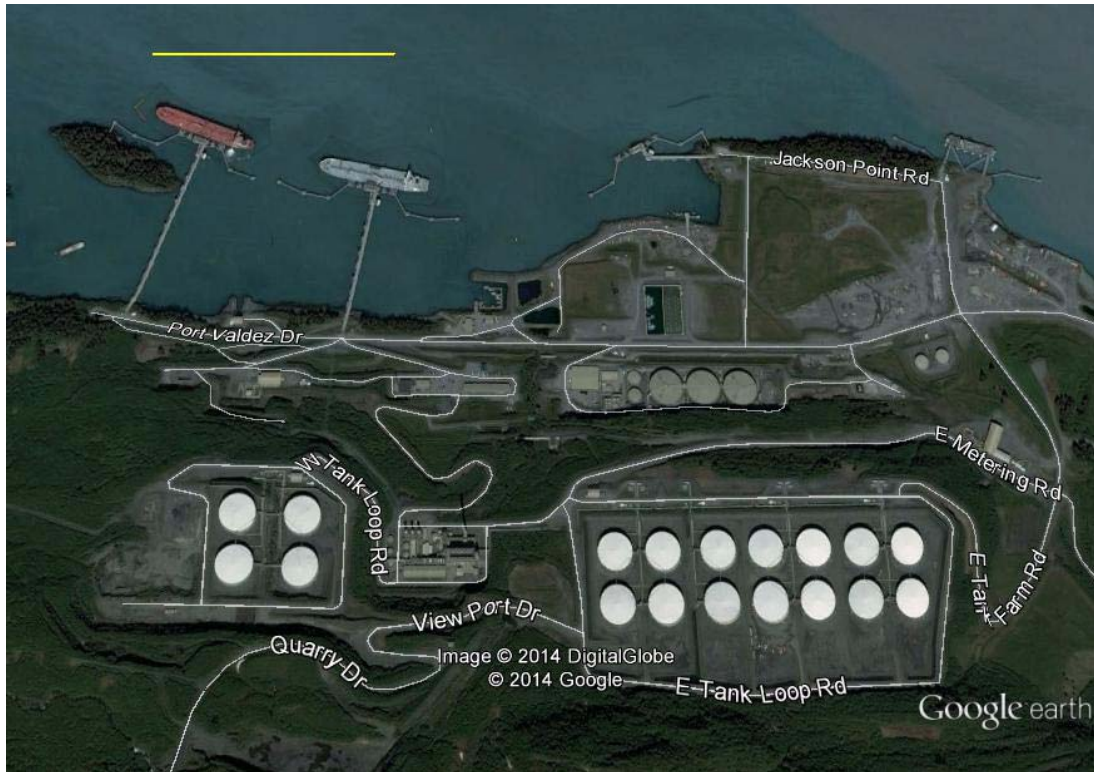
Figure 29 Valdez Terminal – Aerial View
